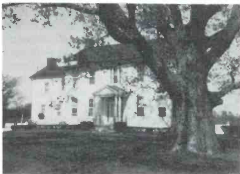
Picturesque former farmhouse serves as FCC Laurel, Maryland monitoring facility. Tree in foreground, one of the oldest in State, reputed to be more than 400 years old.
